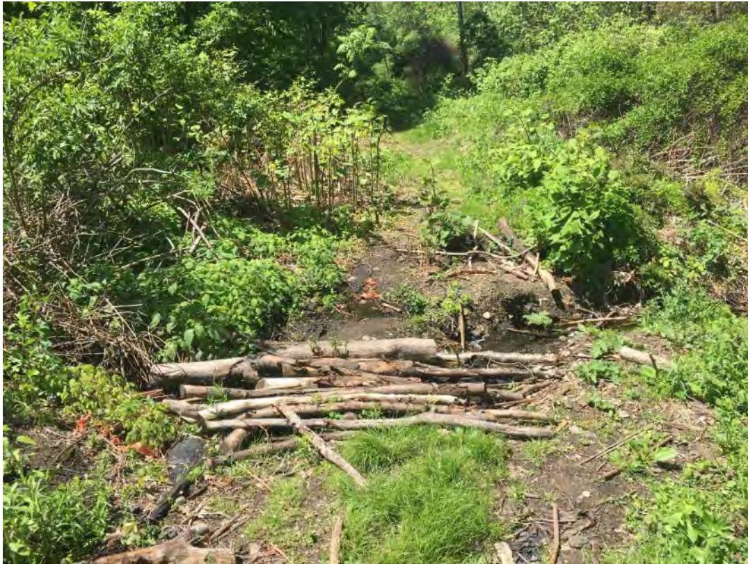
Photo 11. Westerly view of proposed stream crossing at STA 48+00
