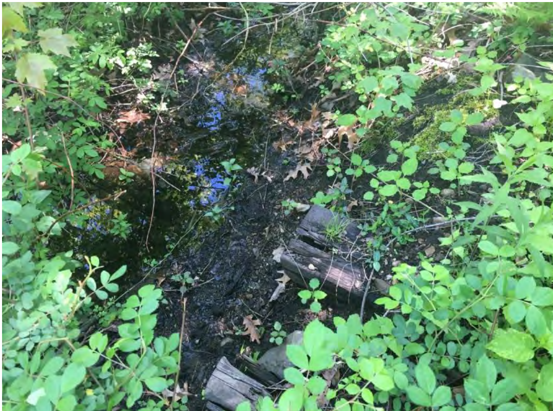
Photo 15. View of existing railroad infrastructure adjacent to existing stream to be relocated.
