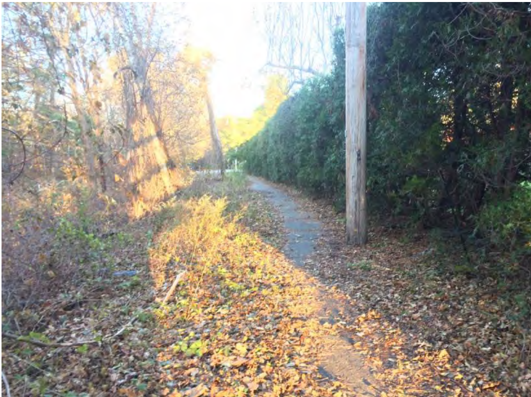
Photo 4. Easterly view of paved path within trail corridor west of Humphrey Street.
