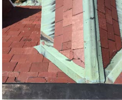
Slate Roof tiles need repair
