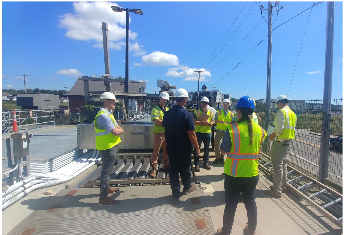
8.31.22 – Site Tour of UV Disinfection System, Newport, RI
