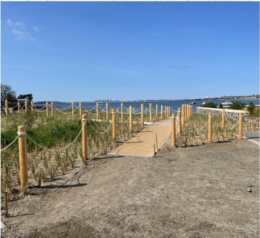
The dune nourishment project at Cassidy Park Beach (below). Highlighted is additional sediment and increased grading of the dune, along with handrails
